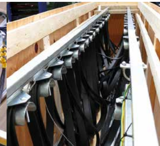
Ready to use hoist power supply
